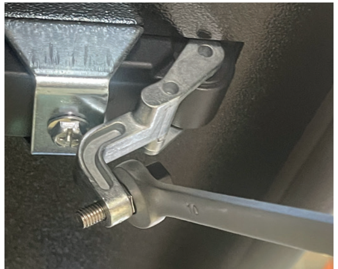
10mm spanner on locking nut
